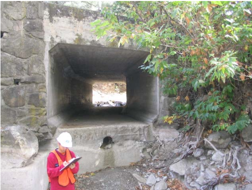
Photo 7. Downstream Face of Culvert, October 2004
