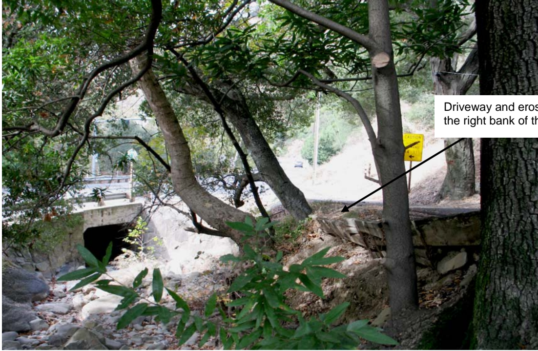
Channel upstream of culvert showing skew of the culvert inlet to the alignment of the channel, the location of the driveway, and the bank erosion along the right bank of the creek.
