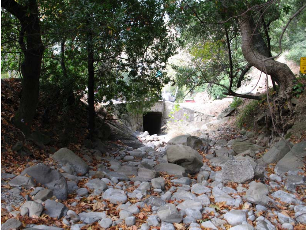
Cobble-boulder substrate of channel upstream of culvert inlet. Channel grade estimated to be 7-8%.
