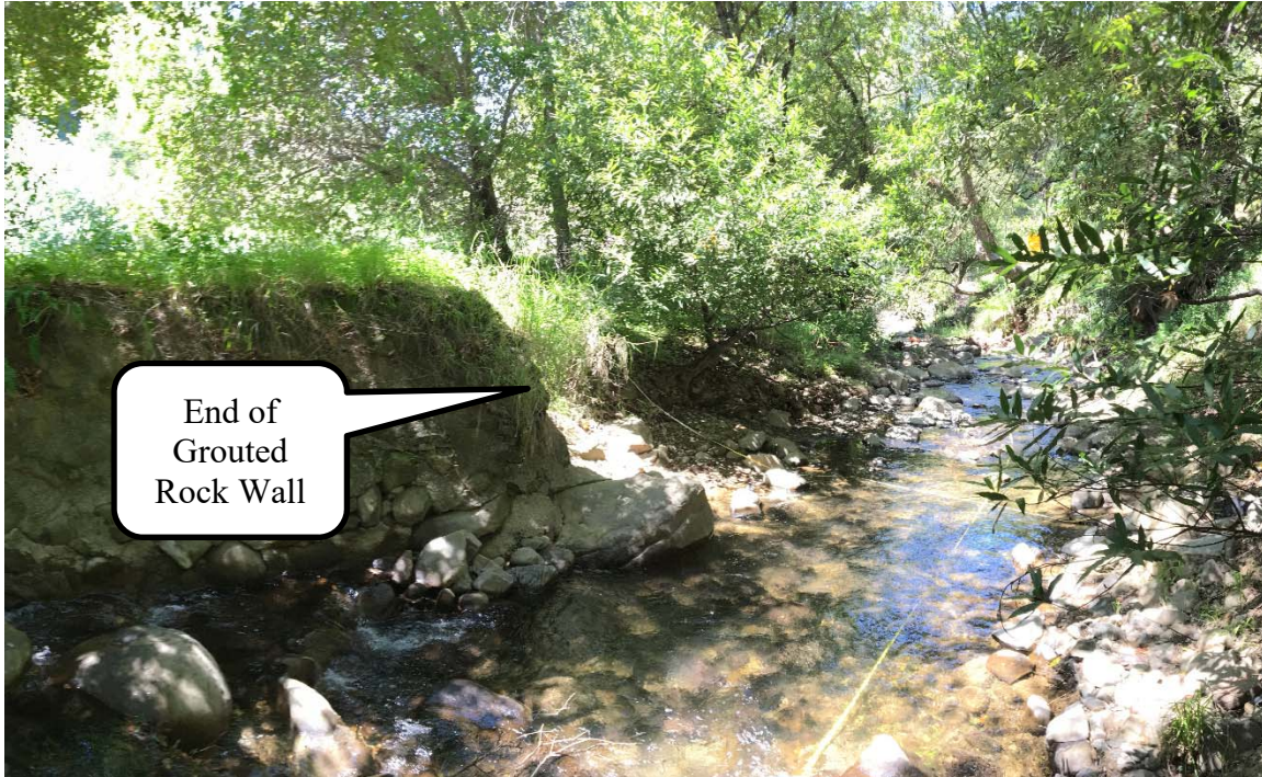
Photo 2. Grouted Rock Wall on Left Bank, Facing Downstream (April, 2019)
