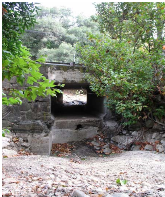
Culvert outlet and downstream scour hole.
