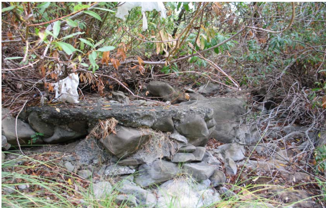
Detail of old crossing remnant on the right bank of Stonybrook Creek at the confluence of Alameda Creek. The crossing element is composed of rock and concrete with asphalt paving on the top surface.
