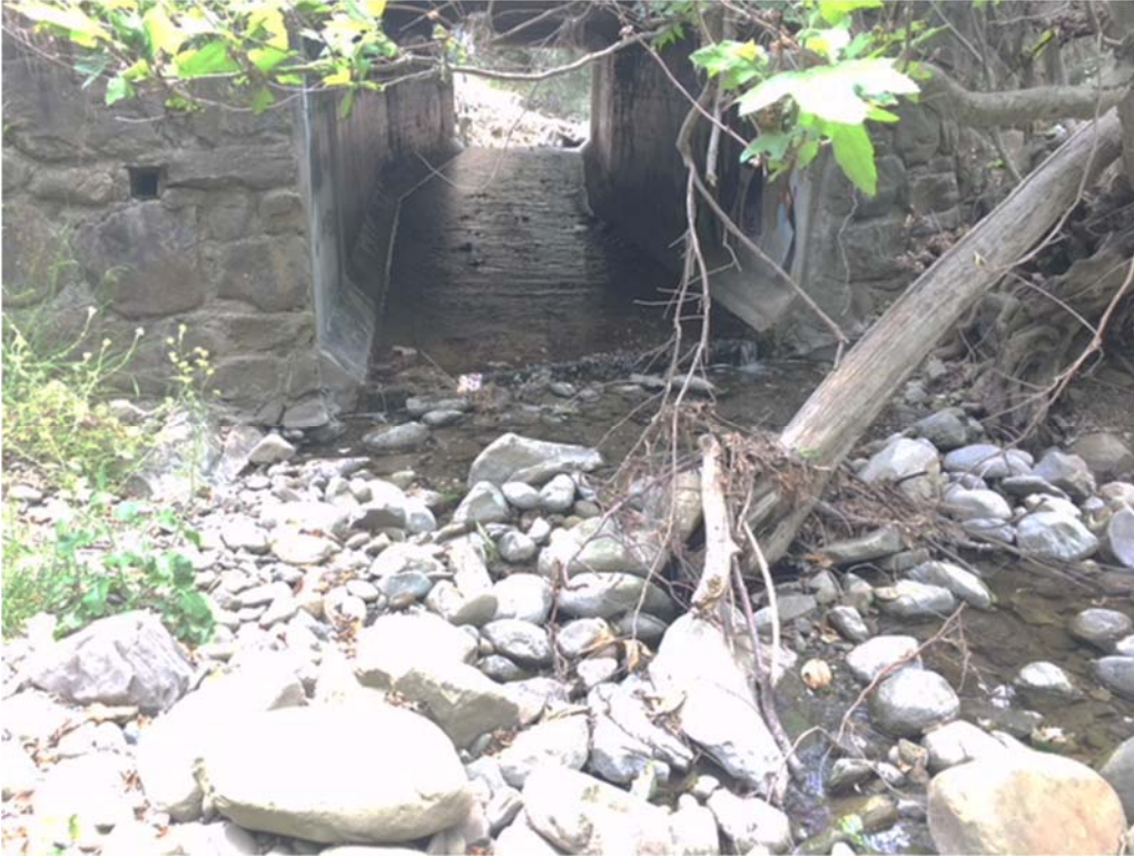
Photo 6. Downstream Face of Culvert, May 2018
