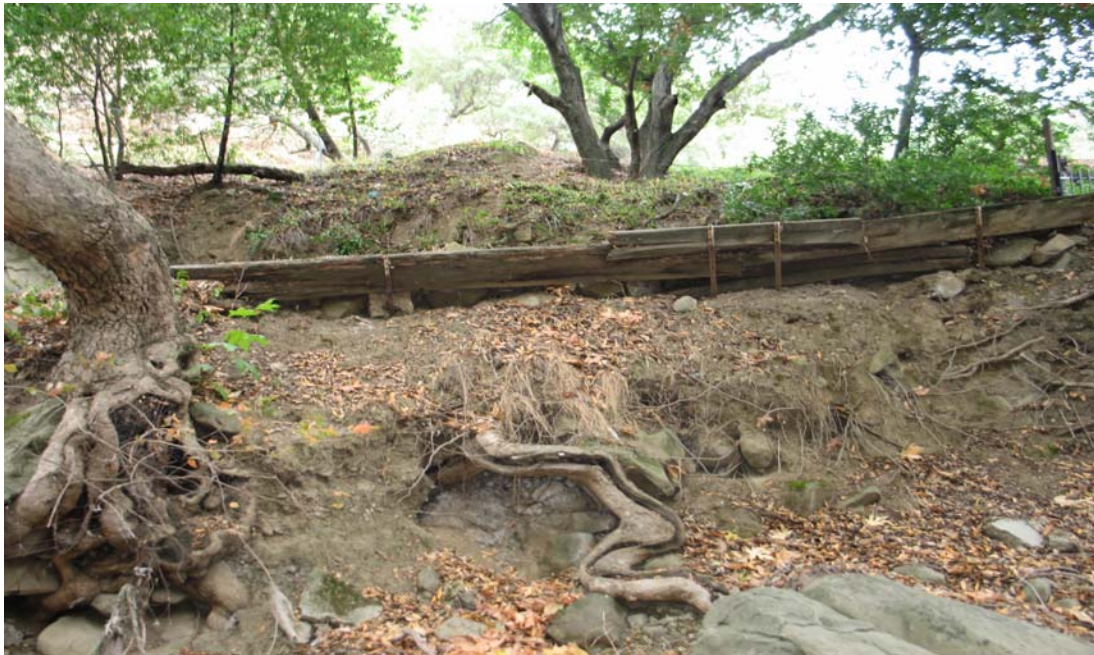
Detail of bank erosion between the driveway and right bank of Stonybrook Creek.
