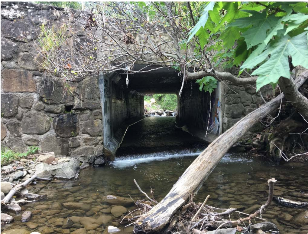
Photo 5. Downstream Face of Culvert, April 2019
