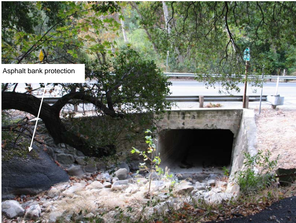
Culvert inlet showing skew of the culvert to the alignment of the channel. Note use of asphalt on the bank at the interface between the bank and left abutment of the culvert.
