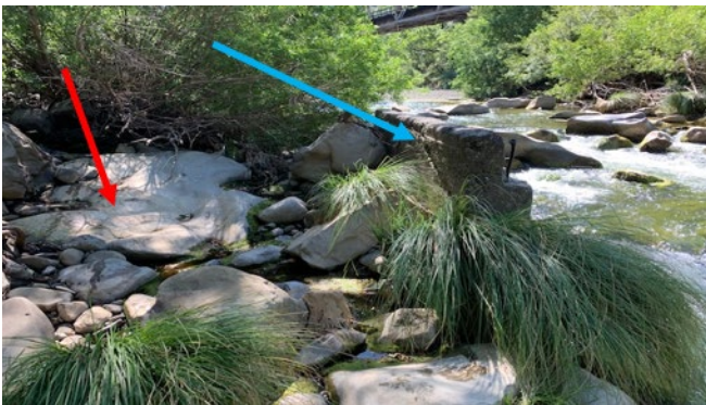
View upstream along Alameda Creek showing old abutment (blue arrow) and large rock formation (red arrow)
