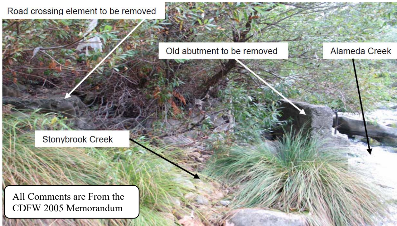
Photo 9. Photo and Comments of the Old Road Remnant and Abutment from the CDFW Memo (2005) (facing upstream)
