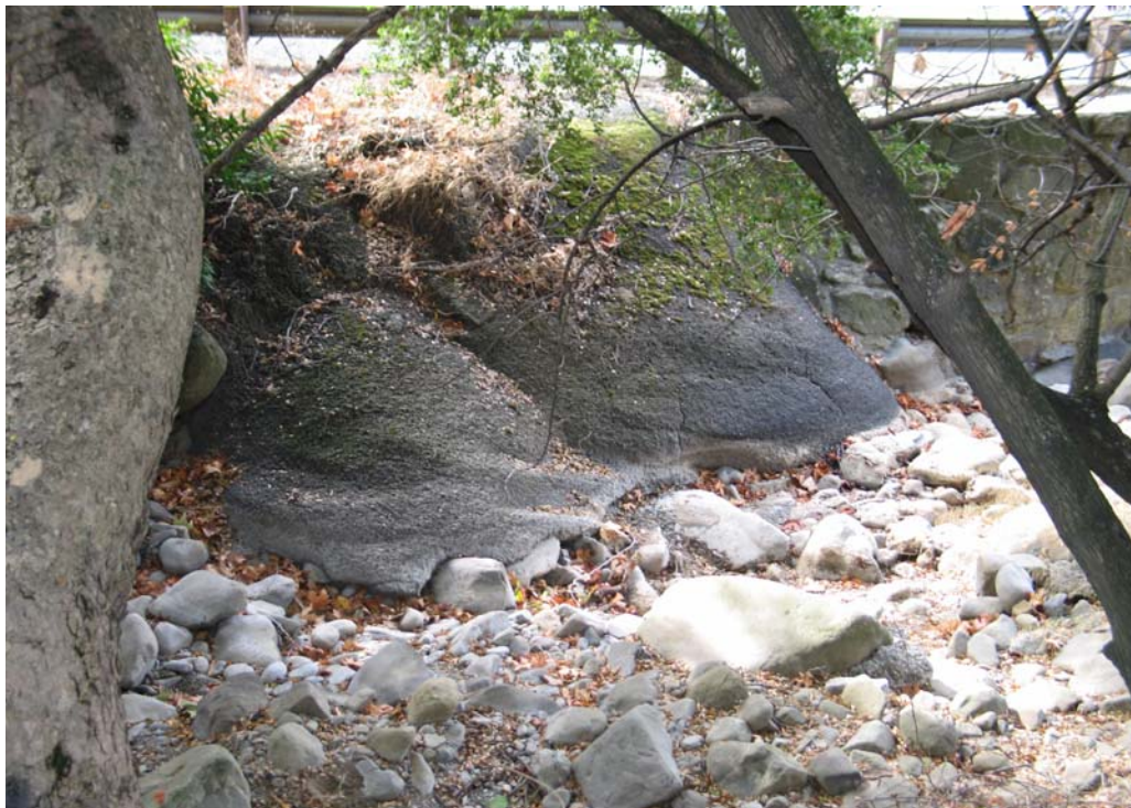
Detail of asphalt bank protection used on the left bank of the creek.
